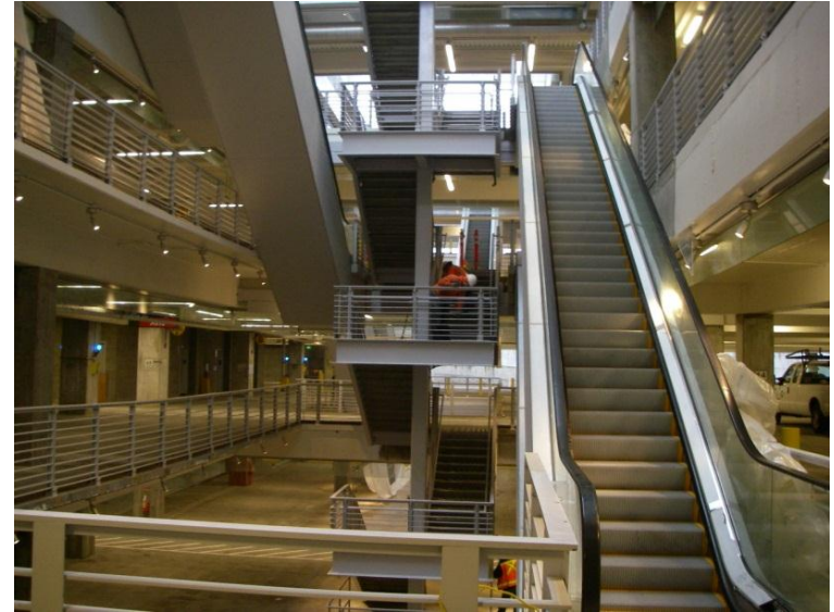
RCF Stair K and Escalator Core
