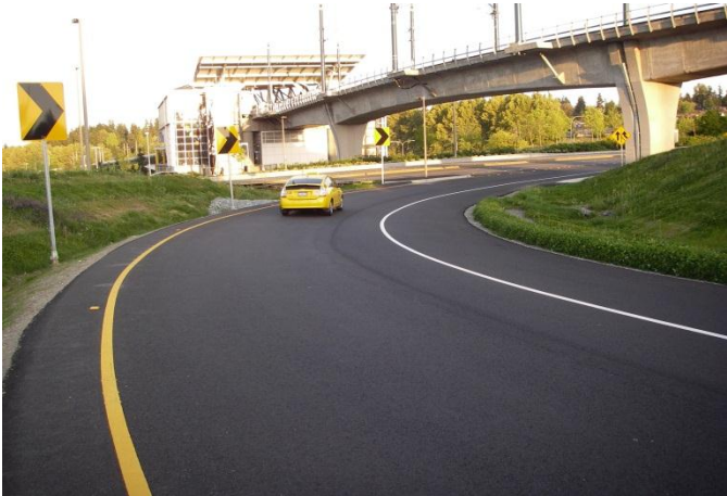
New off ramp from SR-518 Opens
